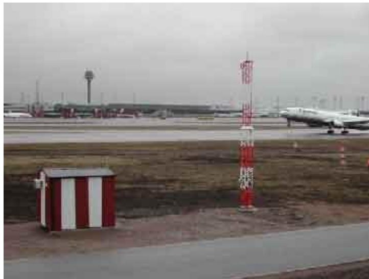
Figure 6-3. The CNS Ground Station and its antenna at Arlanda airport.
