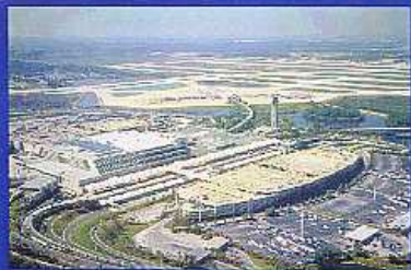
Orlando International Airport
