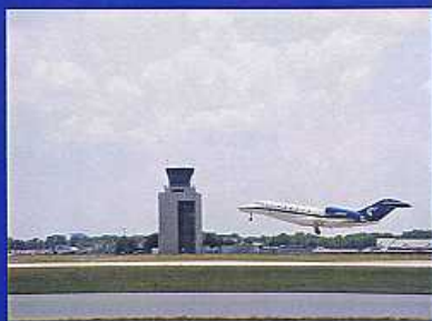
Air Traffic Control Tower Orlando Executive Airport
